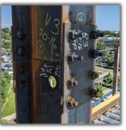
BOLTING INSPECTION Examine structural drawings and plans, confirm proper materials, pre-installation examination, and postinstallation examination.
